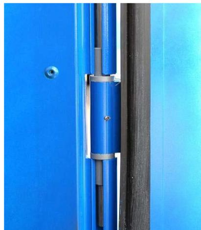
Check hinges for damages and correct operability
